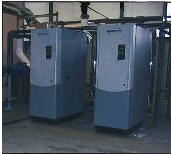
Figure 3-2: CCC Physical Science Building Hot Water Boilers Serving the Hot Water Loop
