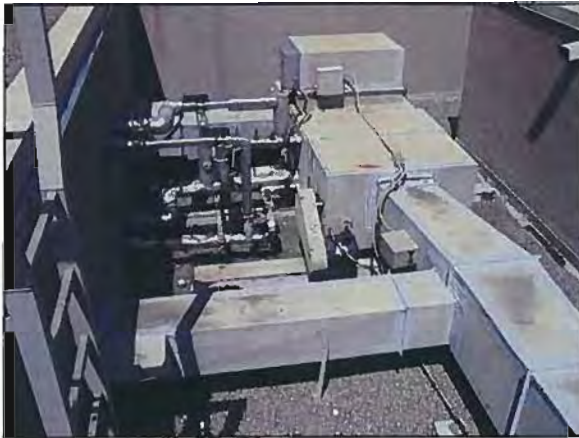
Figure 4-20: CCC Performing Arts Center Rooftop Air Handlers Serving the Preparation Areas
