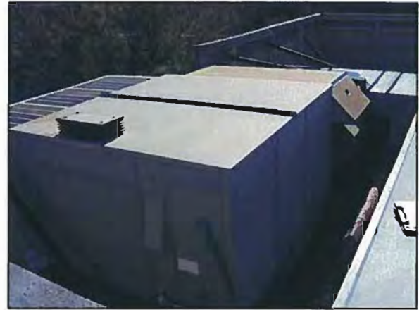
Figure 4-44: Typical Constant Volume Single Zone Unit
