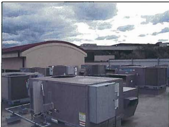
Figure 4-54: LMC Childcare Rooftop Packaged Units
