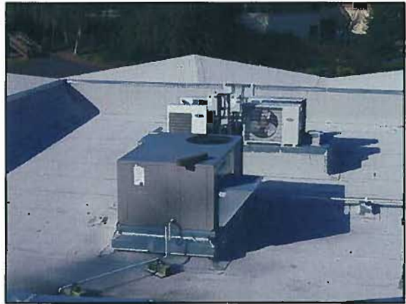
Figures 3-40: DVC Music Building, AC-1 and Heat Pump 1 through Heat Pump 4
