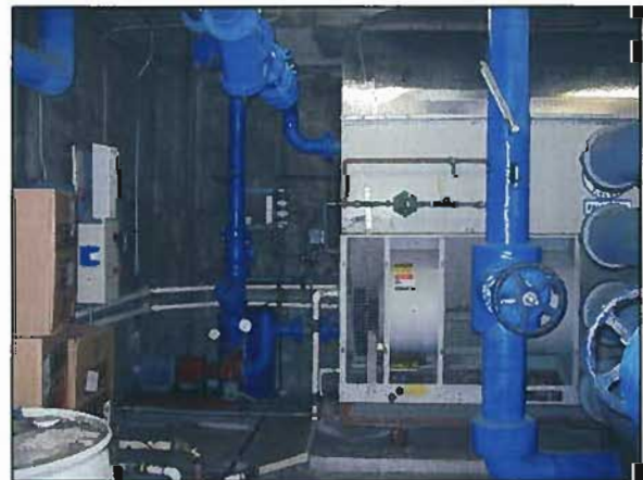
Figure 3-95: District Office Building Cooling Tower and Condenser Water Pump
