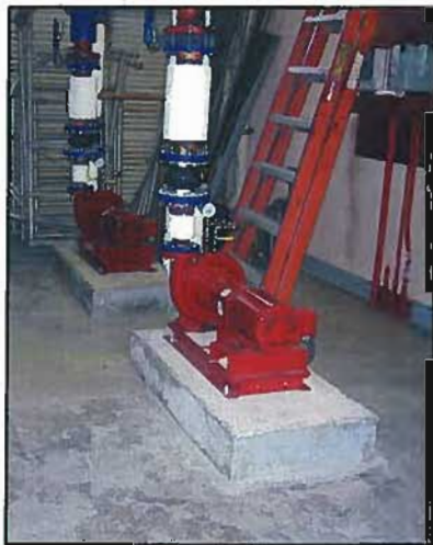
Figure 3-4: Heating Water Pumps Serving the Hot Water Loop
