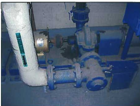
Figure 3-18: CCC Performing Arts Center Chilled Water Pump
