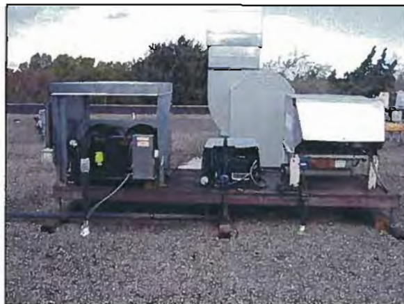
Figure 4-55: LMC Cafeteria Rooftop Packaged Units
