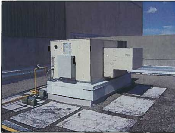
Figure 4-70: One of Eight Packaged Gas/DX Units Serving the LMC Music Addition Building
