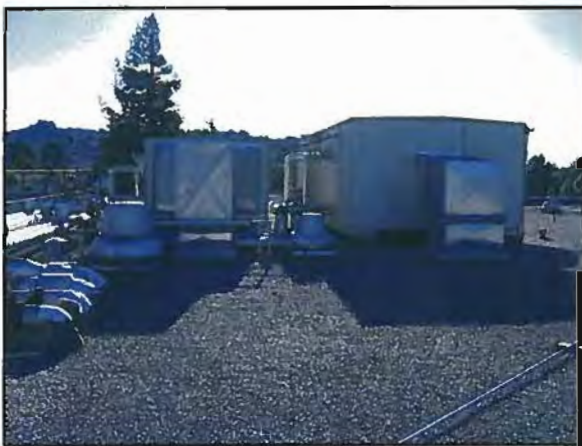
Figure 3-13: Two of Seven Air Handlers in the CCC AA Building
