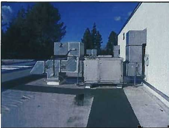
Figures 3-64: DVC Library Building, Typical Reznor Outside Air Supply Fan for Fan Coils
