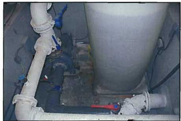
Figure 3-82: LMC Pool Pump
