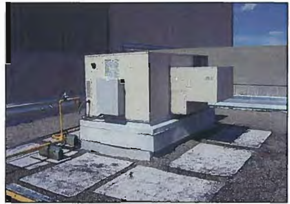
Figure 4-68: LMC Supply Fan Motor Installed on Air Handler; Motor Is 5 or 6 Years Old.
