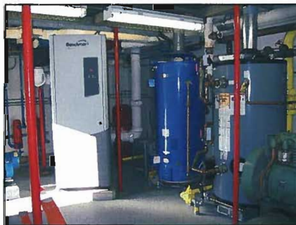
Figure 3-9: CCC AA Building Hot Water Boiler and Domestic Hot Water Heaters
