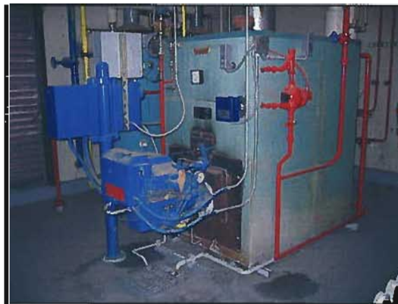
Figure 3-16: CCC Performing Arts Center Gas-Fired Hot Water Boiler
