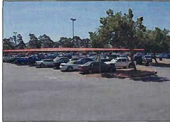
Figure 4-2: Parking Shade Structure
