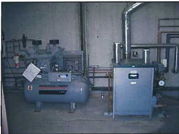
Figure 3-77: LMC Steam Boiler Serving the Science Labs
