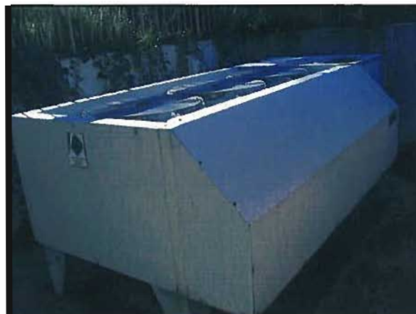
Figure 3-33: DVC Music Building Air-Cooled Chiller
