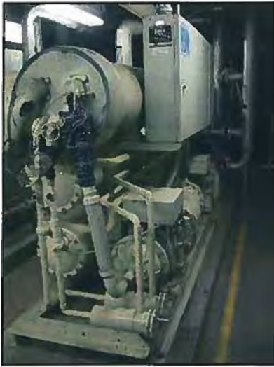
Figures 3-55: DVC Library Building Water-Cooled Chiller
