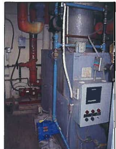
Figure 4-79: District Office Gas-Fired Hot Water Boiler and Water Pump
