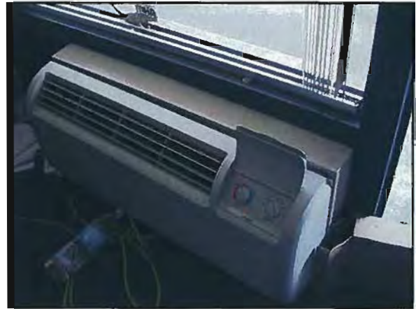
Figure 3-67: DVC Library Building, Typical Window Unit in Office
