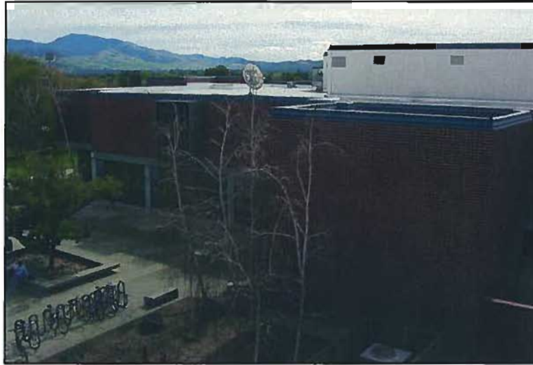
Figure 3-54: DVC Library Building
