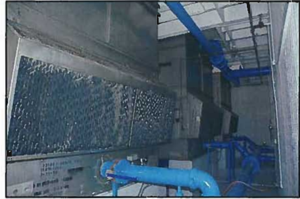
Figure 3-74: LMC Cooling Tower
