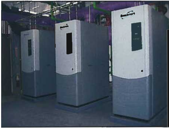
Figure 3-75: LMC Heating Hot Water Boilers
