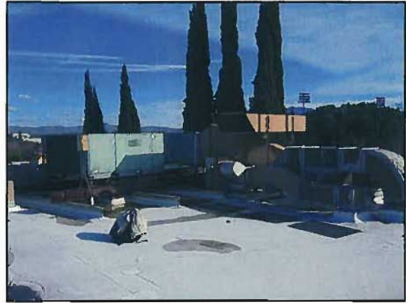
Figures 3-38: DVC Music Building, Old Packaged Rooftop Units AC-4 and AC-5
