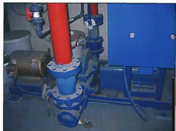
Figure 3-19: CCC Performing Arts Center Condenser Water Pump
