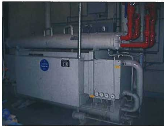
Figure 3-17: CCC Performing Arts Center Water-Cooled Screw Chiller
