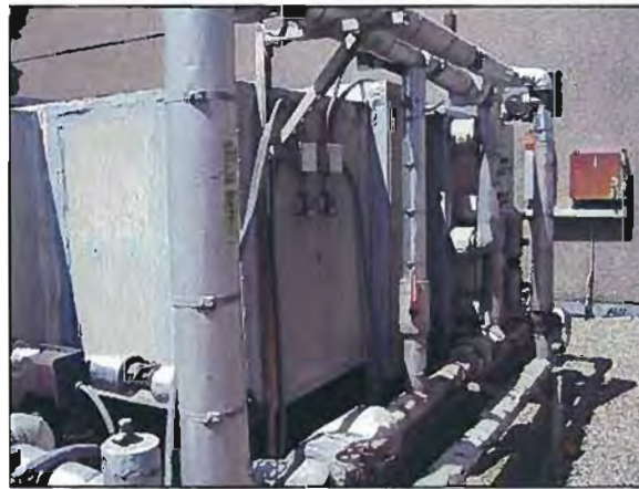
Figure 4-22: CCC Performing Arts Center Air Handler Serving the Theater
