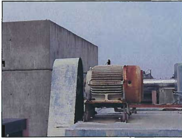
Figure 4-67: LMC Supply Fan Motor Installed on Air Handler; Motor Is 5 or 6 Years Old.
