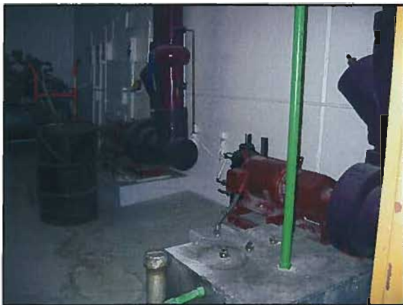
Figure 3-81: LMC Central Plant Chilled Water Pumps
