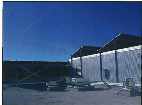
Figure 3-31: DVC Life Health Science Building, Typical Condenser Unit for Split Systems
