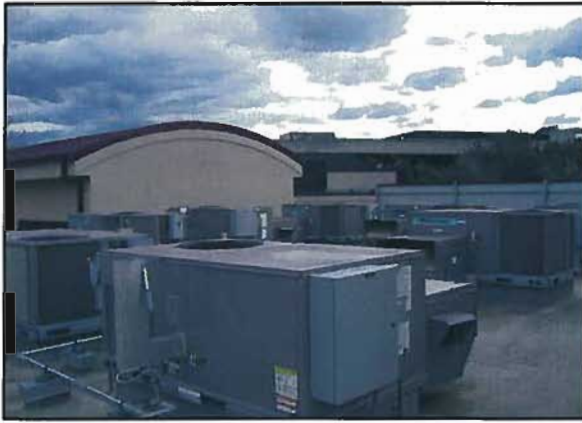
Figure 3-84: LMC Packaged Units on the Roof of the Childcare Center
