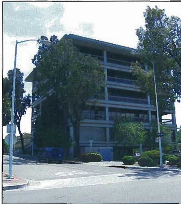
Figure 3-90: District Office Building
