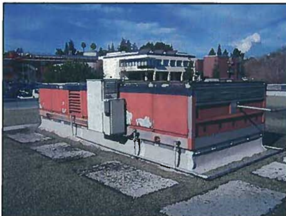
Figure 3-42: DVC Engineering Technology Building, Typical Multi-zone Rooftop Unit with VFD
