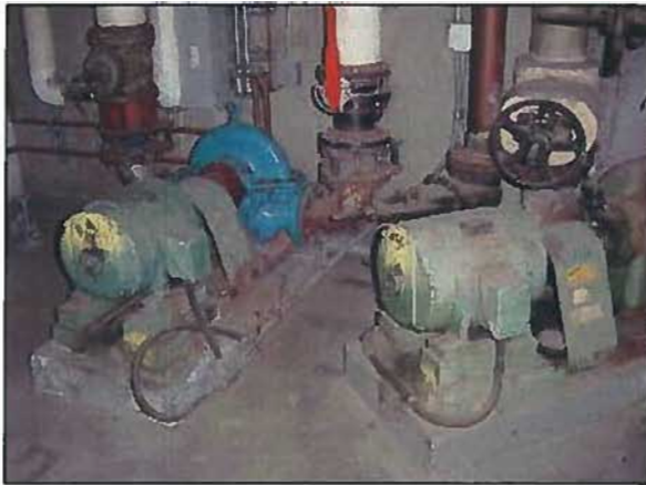
Figure 4-38: DVC Library Building Chilled Water Pump
