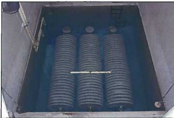
Figure 4-58: LMC Existing DE Filter
