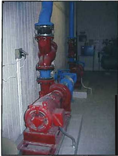
Figure 3-79: LMC Central Plant Condenser Water Pumps
