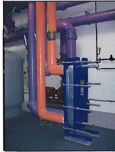
Figure 3-76: LMC Heating Water to Domestic Hot Water Heat Exchanger
