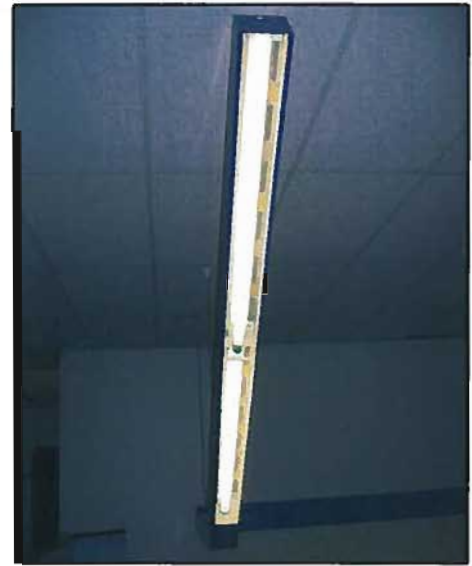
Figure 3-8: CCC AA Building T12 Hallway Lamps
