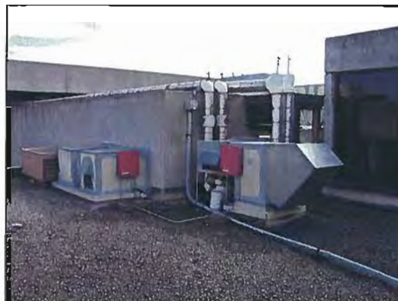
Figure 4-66: LMC Economizer Retrofit on Unit S-8 Where Outside Dampers Are Manually Shut
