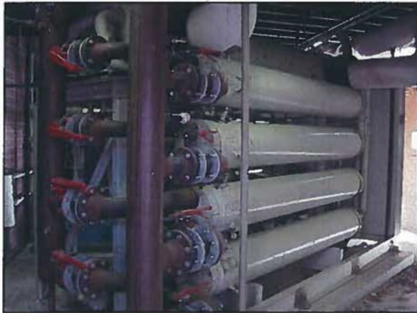
Figure 4-41: DVC Life Health Science Building Water-Cooled Chiller
