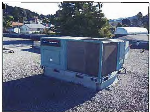
Figure 4-6: CCC Applied Arts and Administration Building Packaged Unit on Roof
