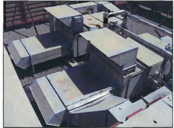
Figure 4-21: CCC Performing Arts Center Rooftop Air Handlers Serving the Preparation Areas
