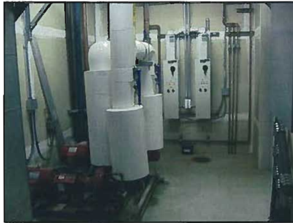
Figure 3-46: DVC Physical Science Building Heating Hot Water Pumps (P-1 and P-2)
