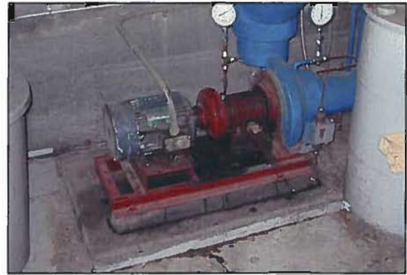
Figure 4-76: District Office Chilled Water Pump
