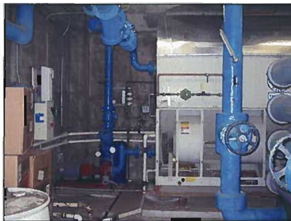
Figure 4-77: District Office Cooling Tower and Condenser Water Pump
