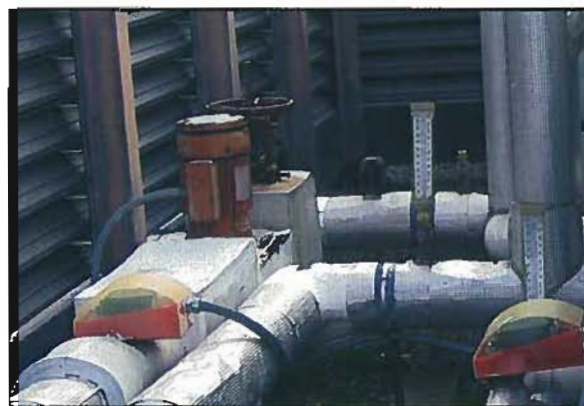
Figure 3-83: LMC Chilled Water Coil Pump
