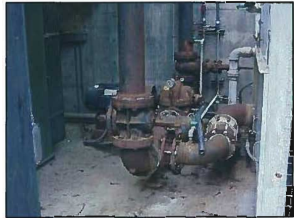
Figure 3-60: DVC Library Building Condenser Water Pump
