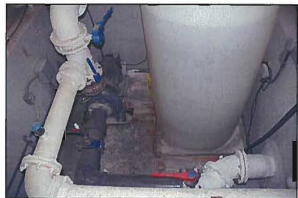
Figure 4-59: LMC Existing Pool Pump
