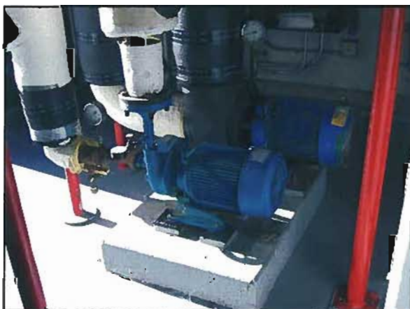
Figure 3-11: CCC AA Building Chilled Water Pumps
