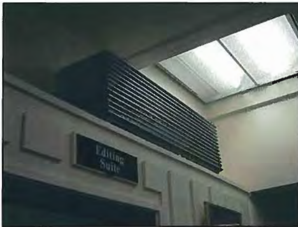
Figure 3-68: DVC Library Building AC Unit for Room L103
