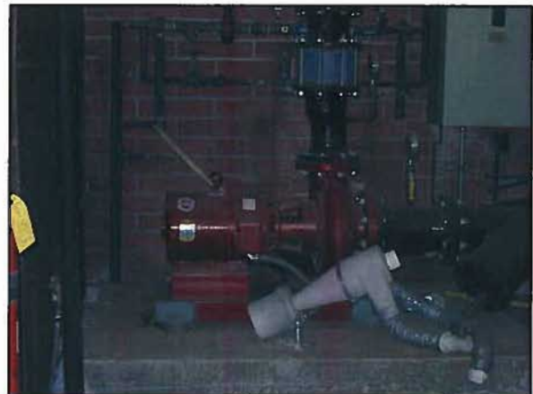
Figure 3-28: DVC Life Health Science Building Condenser Water Pump
