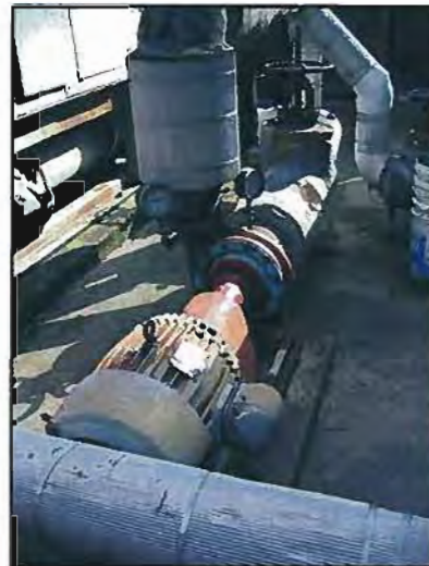
Figure 3-5: CCC Physical Science Building Chilled Water Pump
