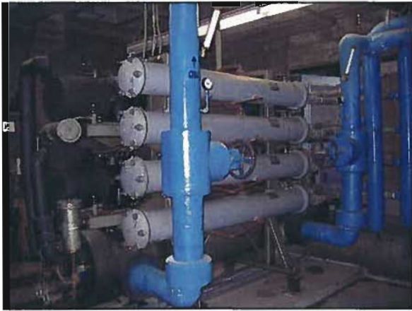
Figure 4-75: District Office Water-Cooled Reciprocating Chiller
