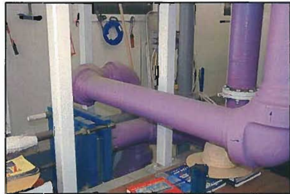
Figure 3-78: LMC Heating Water to Pool Water Heat Exchanger
