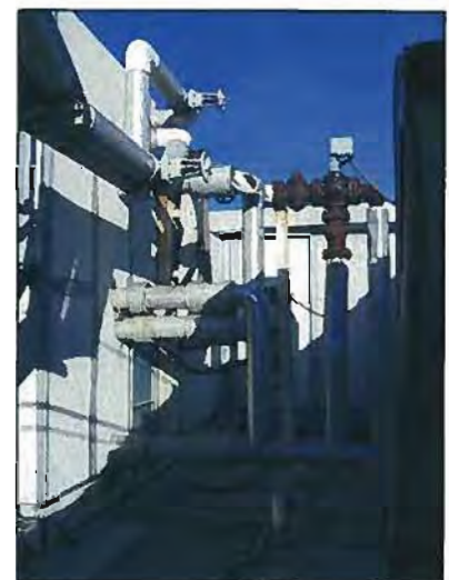
Figure 3-97: District Office Building Rooftop Air Handlers Serving Entire Building
