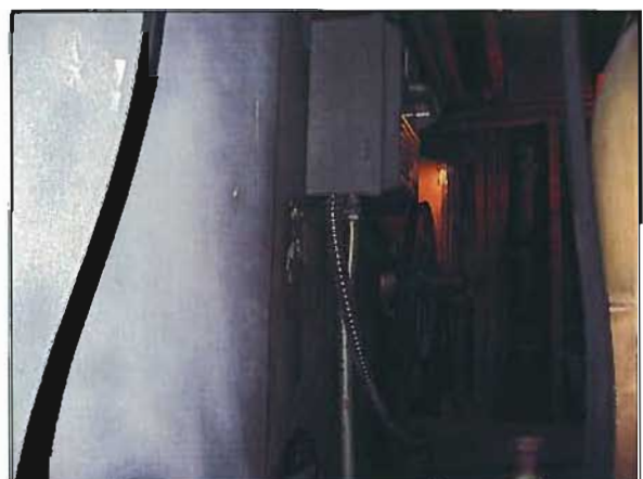
Figure 4-15: CCC Physical Science Building: One of Six Attic Fan Coils Serving the Newer Portion of the Building
