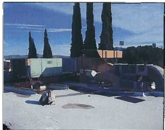
Figure 4-48: DVC Music Building AC-4 and AC-5 Rooftop Units
