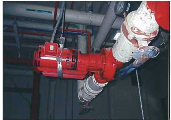
Figure 3-20: CCC Performing Arts Center Hot Water Pump
