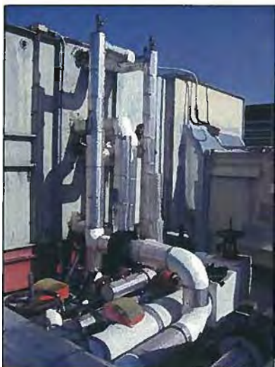
Figure 4-65: Typical Air Handler Located on Roof
