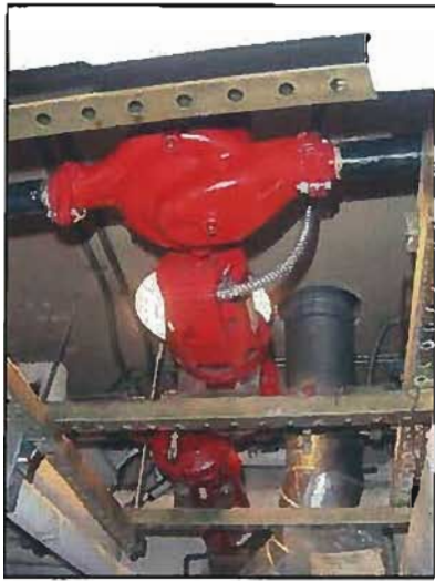
Figure 3-51: DVC Men's Locker Building Heating Hot Water Pumps
