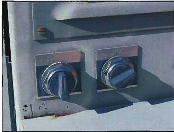
Figure 3-44: DVC Engineering Technology Building VFD Switched to Bypass Mode
