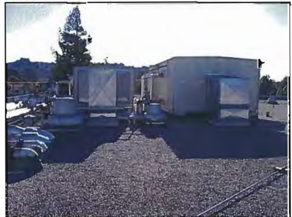
Figure 4-12: CCC Applied Arts and Administration Building Rooftop Air-Handling Units
