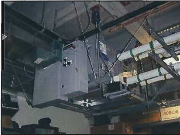
Figure 3-66: DVC Library Building, New Fan Coil Unit FC 1-1 Serving the New Addition on the First Floor
