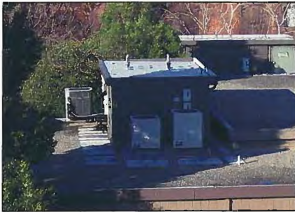
Figure 4-28: DVC Counseling Building Condensing Units on Roof
