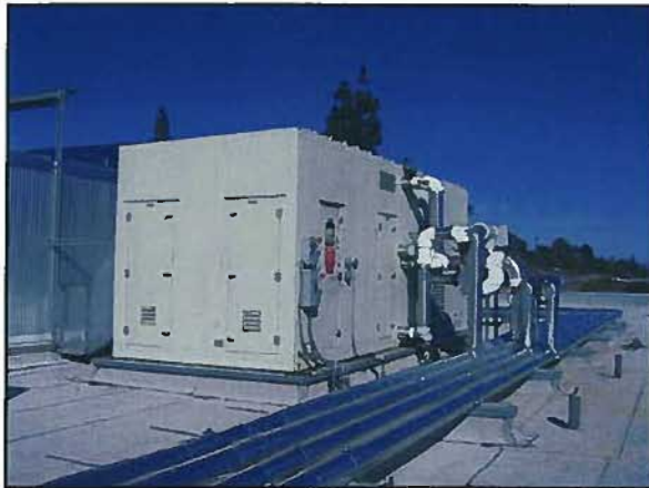
Figure 3-30: DVC Life Health Science Building, Typical Air Handler
