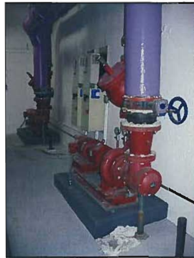
Figure 3-80: LMC Central Plant Heating Water Pumps
