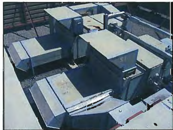
Figure 3-22: CCC Performing Arts Center Rooftop Air Handlers Serving the Preparation Areas
