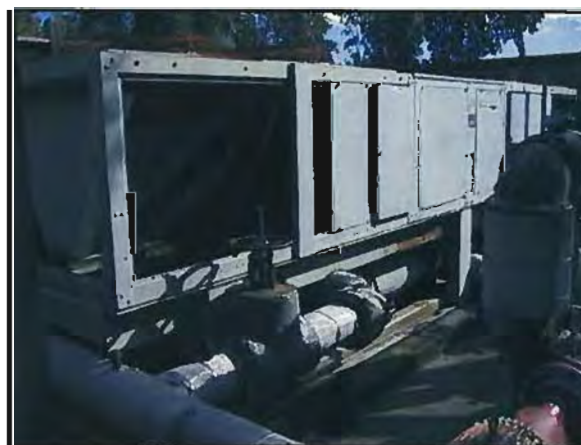
Figure 3-3: CCC Physical Science Building Chiller
