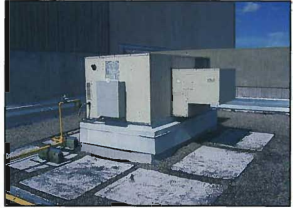
Figure 3-85: LMC Packaged Unit on the Roof of the Music Building
