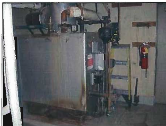
Figure 3-49: DVC Men's Locker Building Heating Hot Water Boiler
