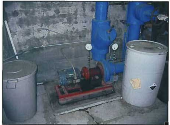
Figure 3-96: District Office Building Chilled Water Pump
