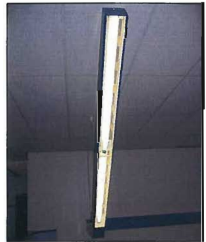
Figure 4-3: Contra Costa College T12 Fixture
