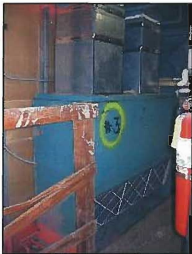
Figure 3-62: DVC Library Building, Typical Fan Coil Unit
