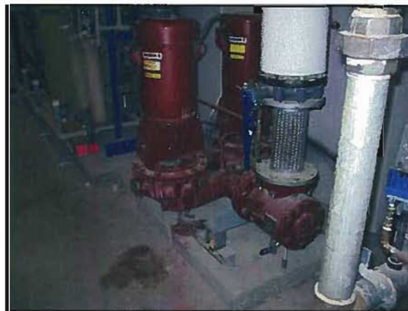
Figure 3-29: DVC Life Health Science Building Heating Hot Water Pumps
