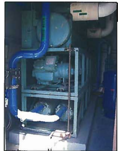
Figure 3-10: CCC AA Building Chiller
