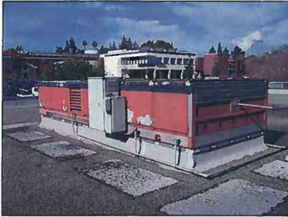
Figure 4-43: Typical Multi-zone Rooftop Unit with VFD
