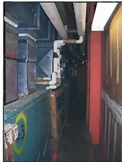
Figure 3-63: DVC Library Building, Typical Fan Coil Unit
