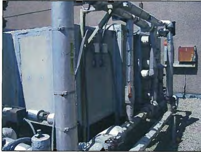
Figure 3-23: CCC Performing Arts Center Air Handler Serving the Theater
