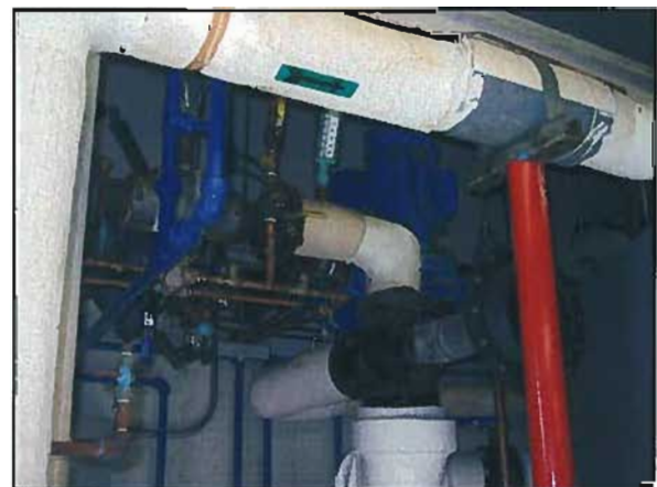
Figure 3-12: CCC AA Building Heating Water Pumps
