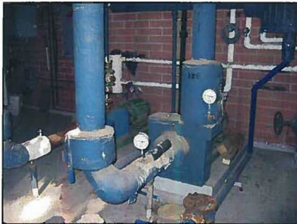
Figures 3-27 DVC Life Health Science Building Chilled Water Pumps
