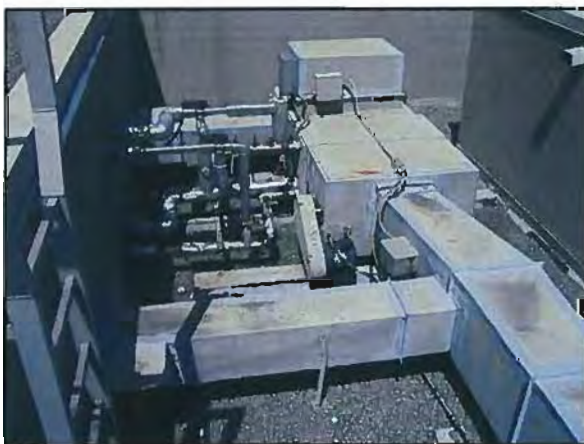
Figure 3-21: CCC Performing Arts Center Rooftop Air Handlers Serving the Preparation Areas
