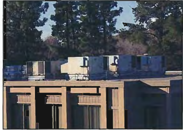
Figure 4-29: DVC Learning Center Condensing Units on Roof
