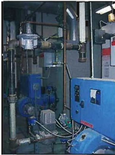
Figure 3-26: DVC Life Health Science Building Heating Hot Water Boiler
