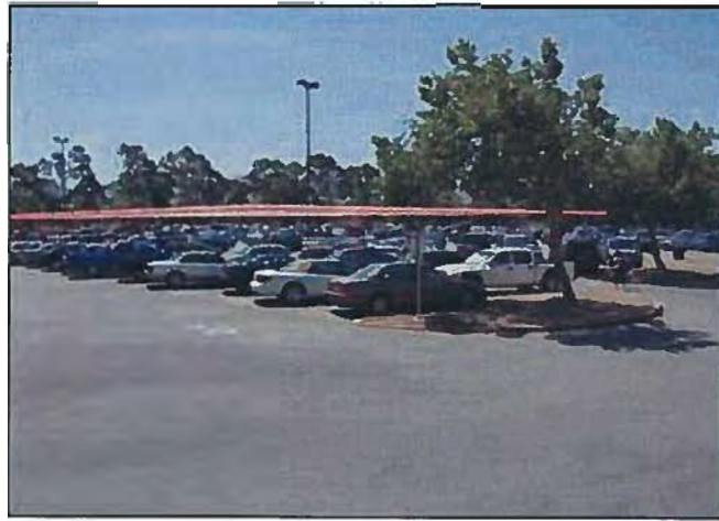
Figure 4-24: Parking Shade Structure
