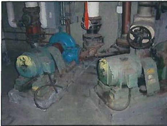
Figure 3-59: DVC Library Building Chilled Water Pump and Heating Hot Water Pumps
