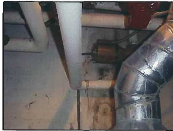
Figure 3-52: DVC Men's Locker Building, Domestic Hot Water Pump
