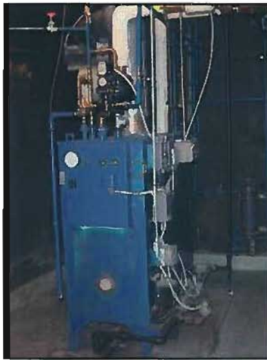
Figure 3-34: DVC Music Building Heating Hot Water Boiler
