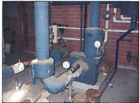
Figure 4-42: DVC Life Health Science Building Chilled Water Pumps
