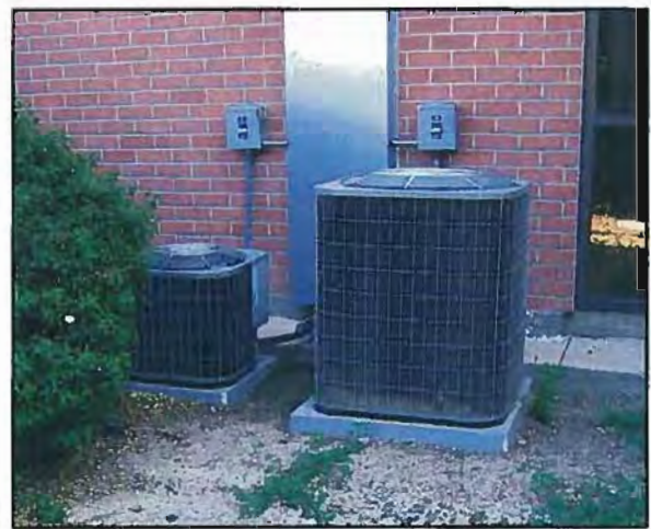
Figure 3-14: CCC AA Building Split-System Condensing Units Serving the Computer Labs
