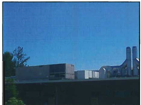
Figures 3-47: DVC Physical Science Building, Typical DX Air Handler
