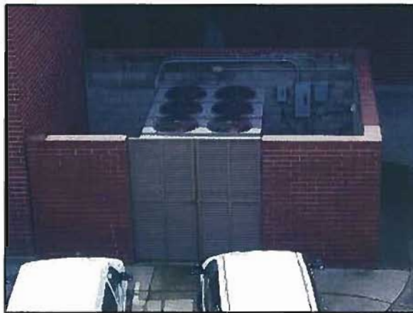
Figure 3-57: DVC Library Building Air-Cooled Chiller for Computer Lab
