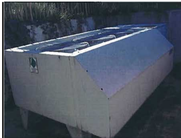
Figure 4-40: DVC Library Building Air-Cooled Chiller
