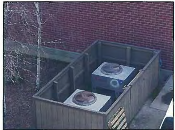
Figure 3-69: DVC Library Building Condenser Units that Serve the Computer Server Room
