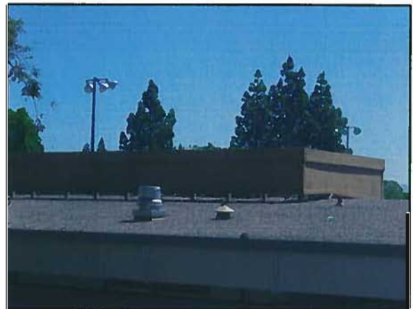
Figures 3-53: DVC Men's Locker Building Fenced Area for Multi-zone Units on Roof
