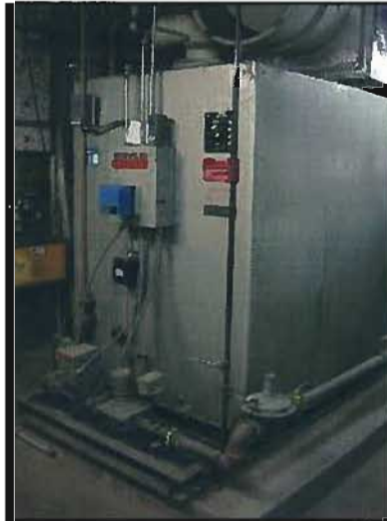
Figure 3-58: DVC Library Building Heating Hot Water Boiler
