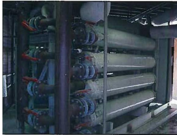
Figure 3-25: DVC Life Health Science Building Water-Cooled Chiller
