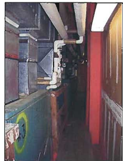
Figure 4-49: DVC Library Building AC Units in Duct Space
