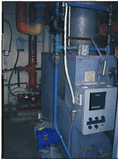
Figure 3-93: District Office Building Hot Water Boiler and Pump
