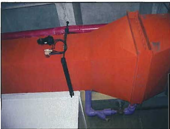
Figure 3-88: LMC VAV Box and Reheat Coil
