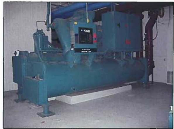
Figure 4-71: One of Two VSD Water-Cooled Chillers at LMC
