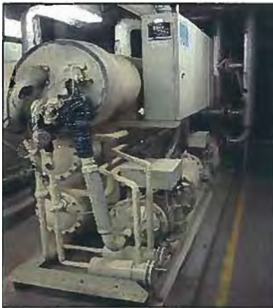
Figure 4-36: DVC Library Building Existing Water-Cooled Chiller
