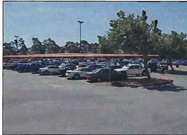
Figure 4-51: Parking Shade Structure
