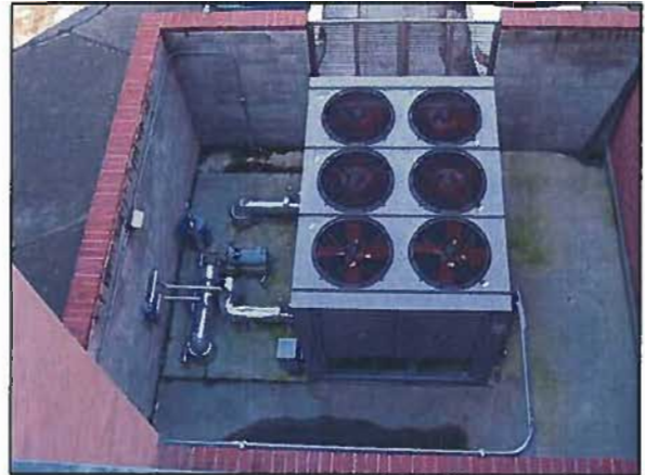
Figure 4-39: DVC Library Building Air-Cooled Chiller
