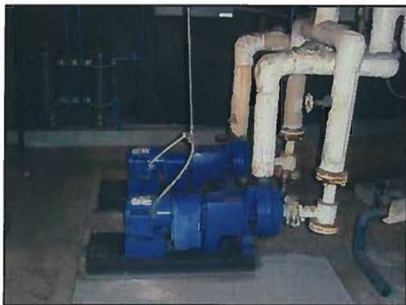
Figure 3-35: DVC Music Building Chilled Water Pumps
