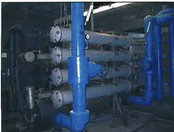
Figure 3-94: District Office Building Chiller
