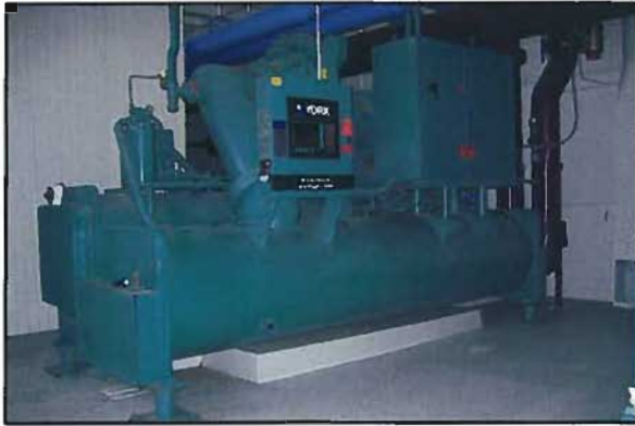
Figure 3-73: LMC Water-Cooled Chiller
