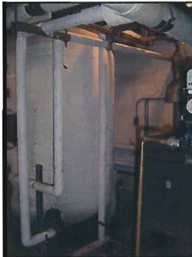
Figure 3-50: DVC Men’s Locker Building Domestic Hot Water Boiler and Hot Water Storage Tank
