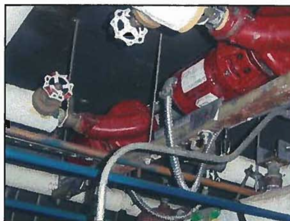
Figures 3-36: DVC Music Building Heating Hot Water Pumps
