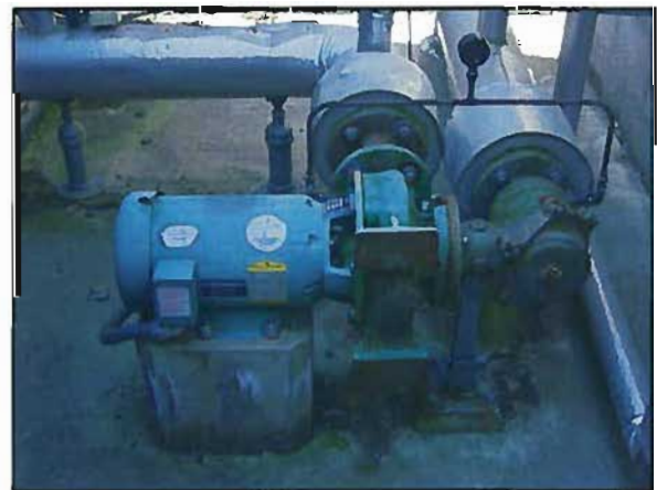
Figure 3-61: DVC Library Building Chilled Water Pump for Air-Cooled Chiller
